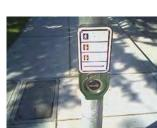
Accessible Path (y/n) YES Clear Floor Space (y/n) YES Clear Floor Slope (%) 1.6 Clear Floor X Slope (%) 1.9 Button Ht. (in) 42 **Button Reach** (in) 0 **Button Diameter** (in) 3 **Button Pressure** (lbs) 1 **Closed Fist Operation** (y/n) YES Visual Contrast (y/n) YES Contrasting Color Bands (y/n) NO Audible Walk Indicator (y/n) YES **Button Locator Tone** (y/n) YES
