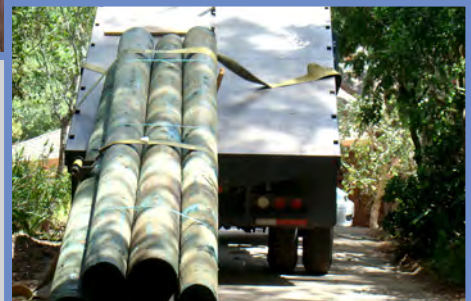
BEFORE - driveway falling downhill
