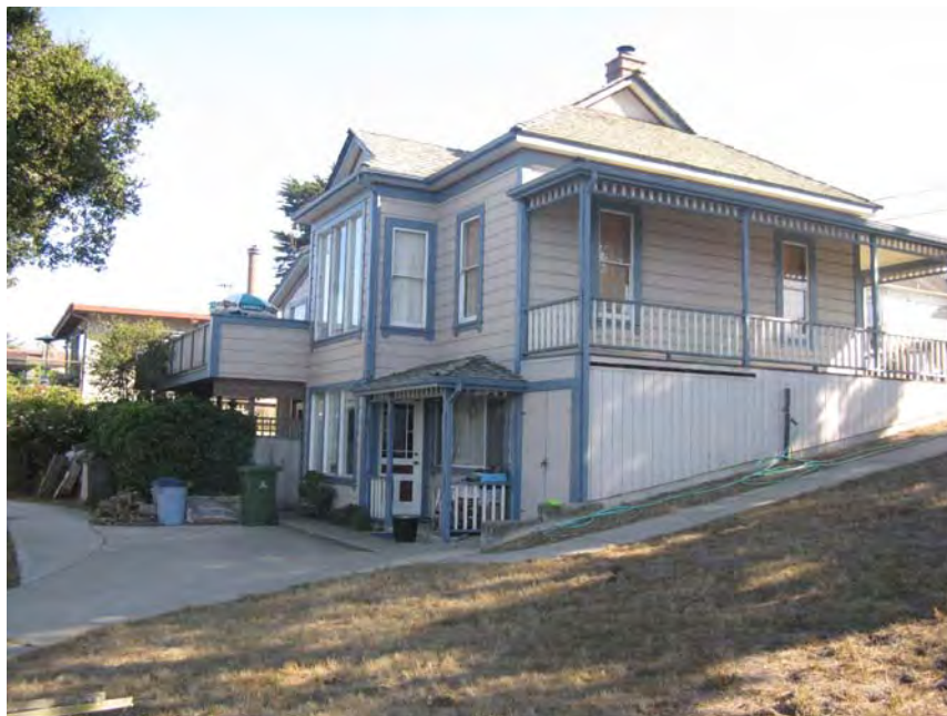
Detail of the north and east (rear) facades from Prescott Avenue (Page & Turnbull)
