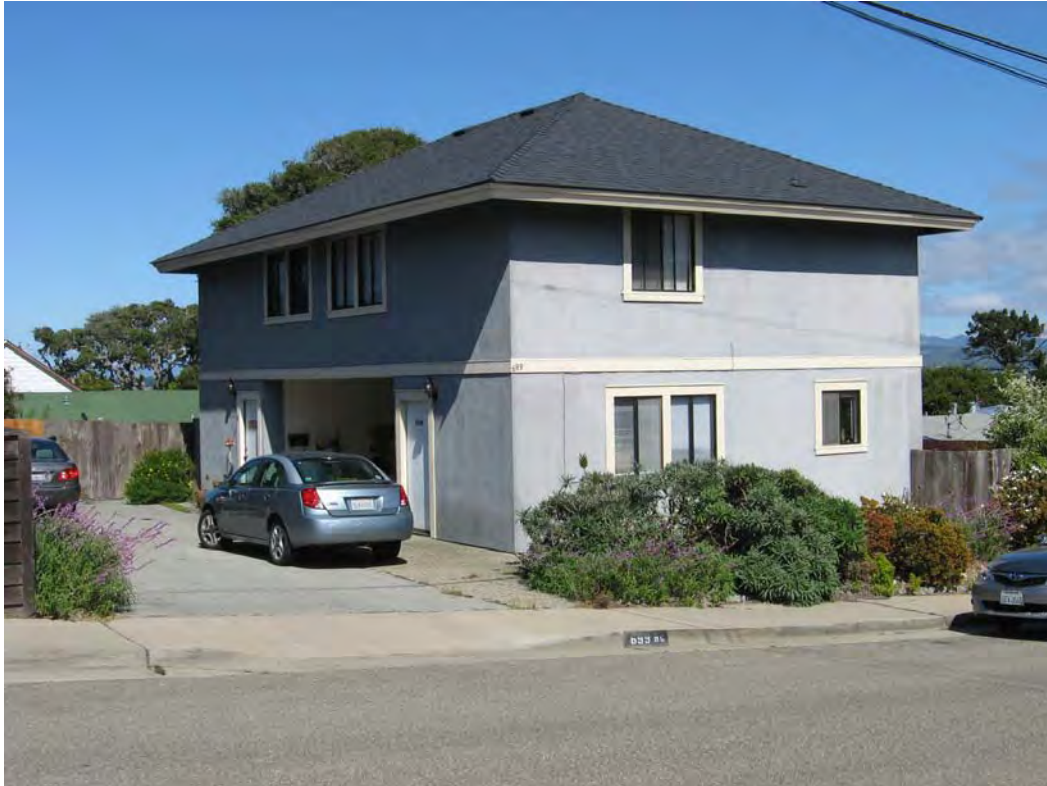
Front (northwest) and southwest façades of 699 B & C David Avenue
