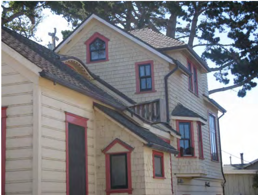
Detail of east facade with rear addition (Page & Turnbull)
