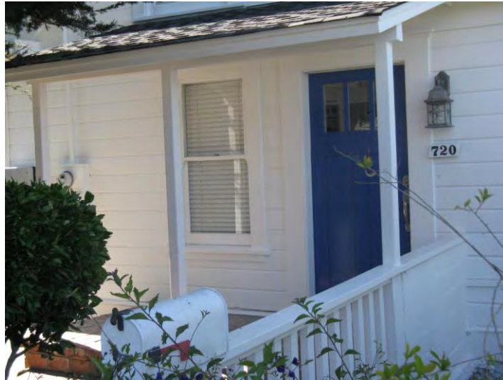
Detail of primary entry on the south facade (Page & Turnbull)
