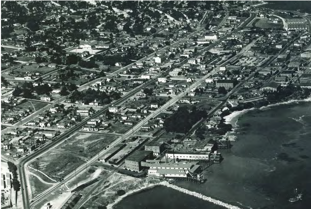
Figure 8-2. Early 1940s aerial of New Monterey, looking northwesterly (courtesy Monterey Public Library, California History Room).
