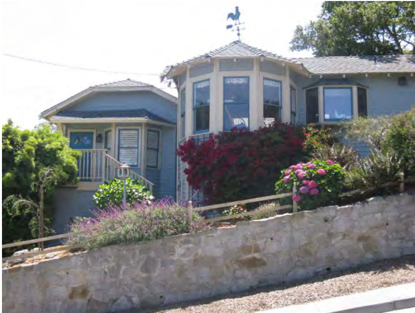
Detail of the north facade from Prescott Avenue (Page & Turnbull)
