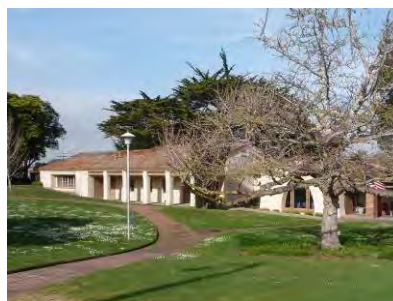
Scholze Park Center 321 Foam Street (1931 portion)
