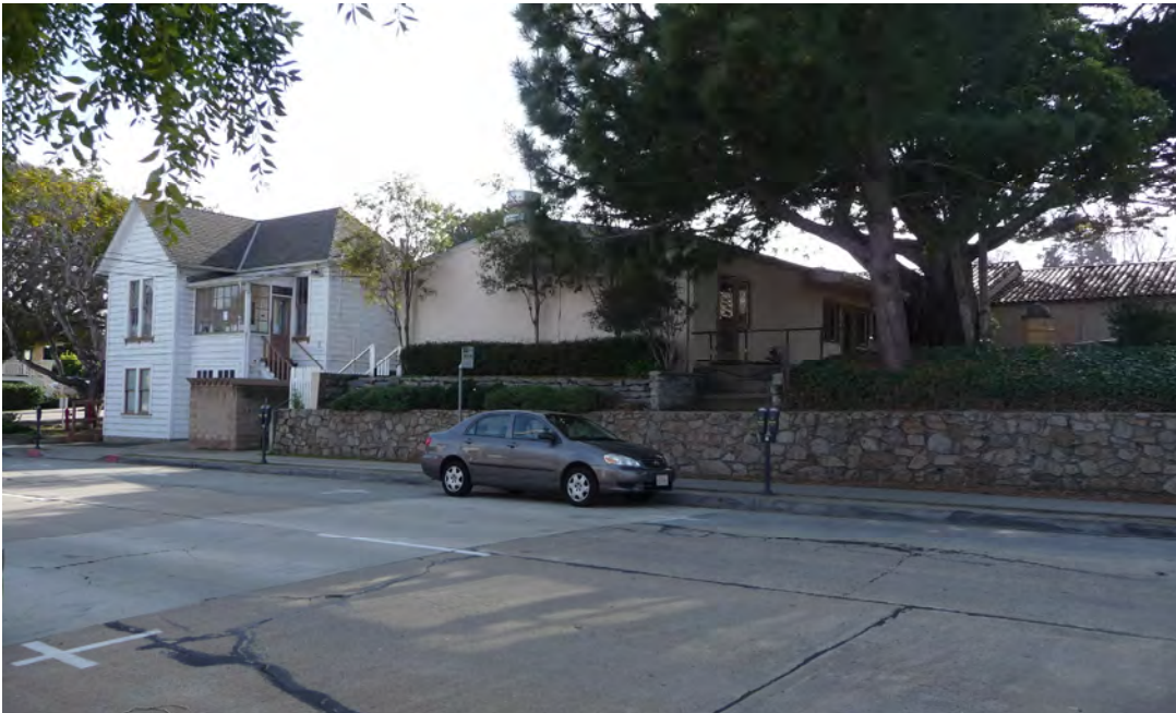
View of east and north elevations (ARG, February 21, 2012).
