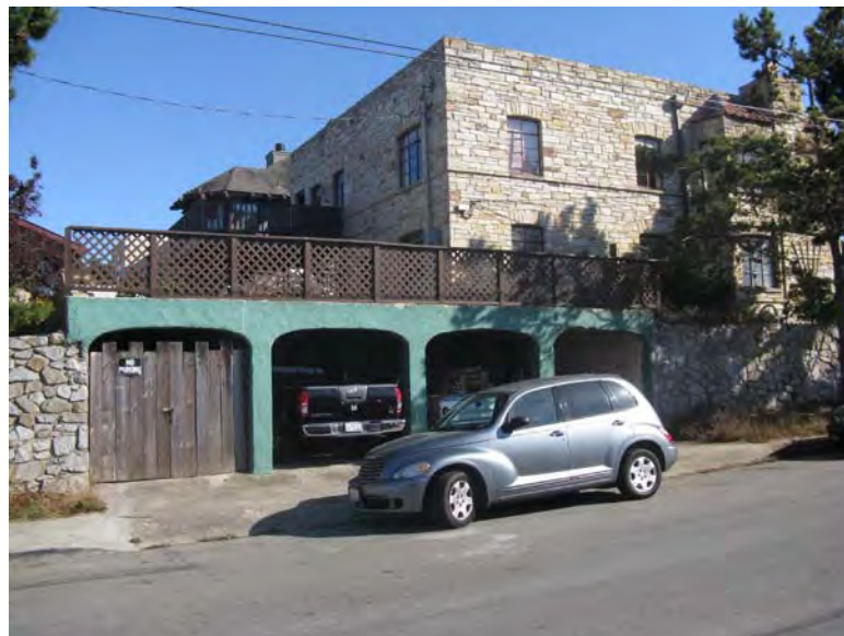
Detail of the north and rear facades from Irving Avenue (Page & Turnbull)
