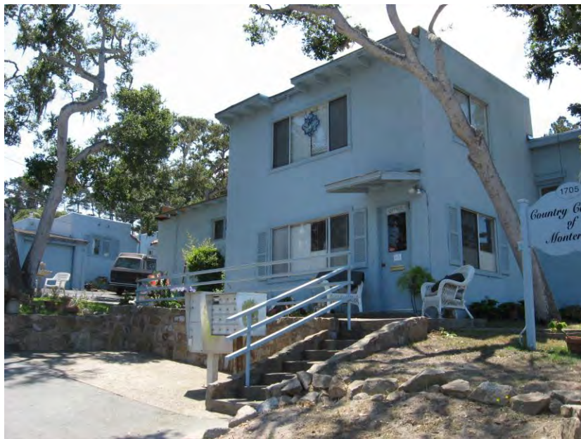
Two-story office building at north corner of lot, looking south from David Avenue.
