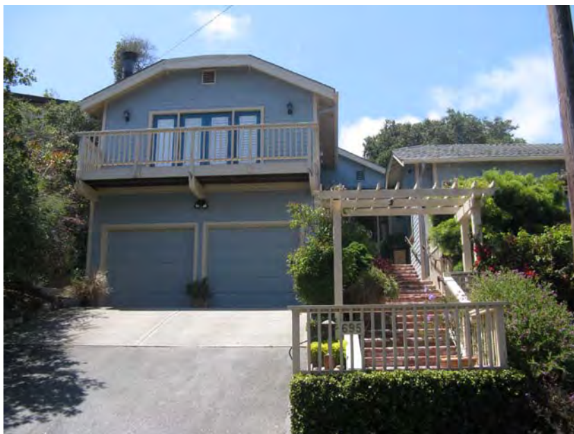
Detail of the east facade from Grace Street (Page & Turnbull)
