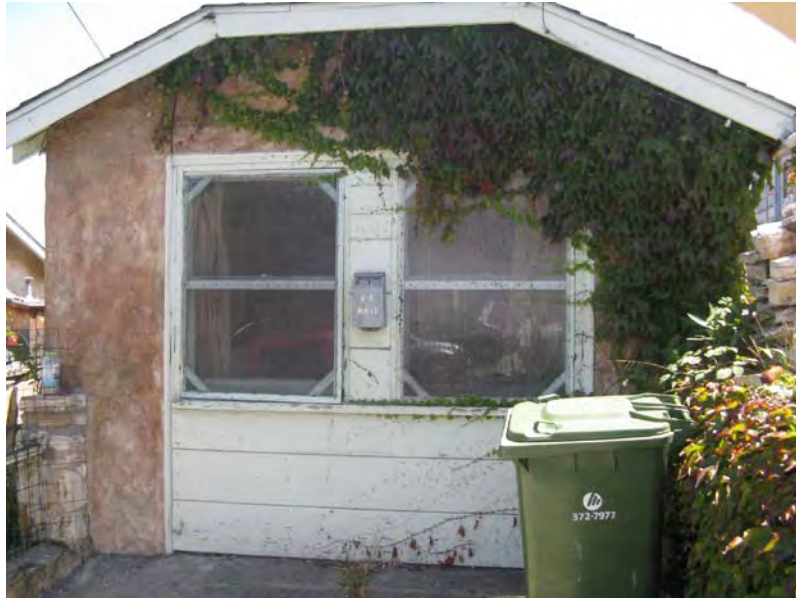
Front (northwest) façade of 509 ½ David Avenue
