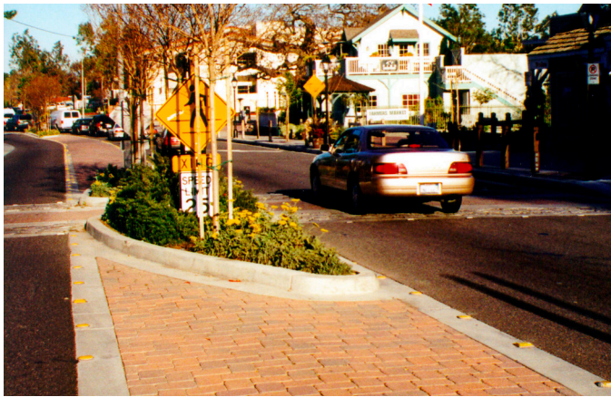
Example of a raised island in center of roadway which incorporated a change in paving and traffic signage to slow down traffic
