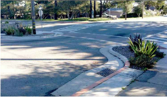
Example of a bulbout that narrows the roadway and shortens pedestrian crossings
