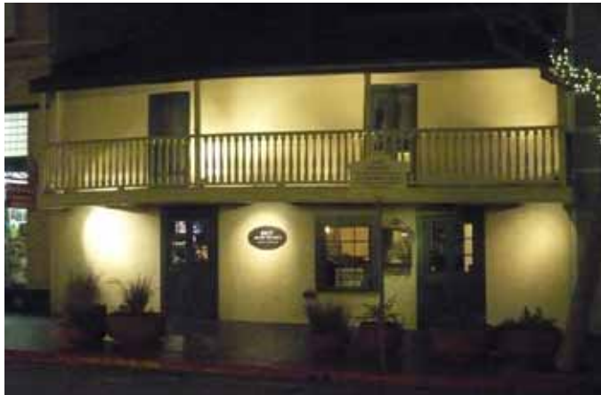
Low level, concealed lighting on historic adobe structures should be encouraged.
