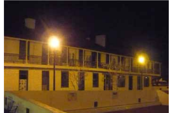
Fixtures in the Heritage District have sodium lamps, which do not complement the character of the buildings in the area.
