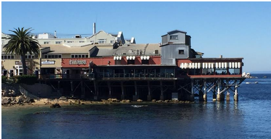
Figure 6-1: Fish Hopper Restaurant (1-2 stories) supported on Open Pile Foundation
