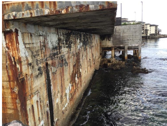
Figure 6-7: Monterey Bay Inn Seawall / Foundation
