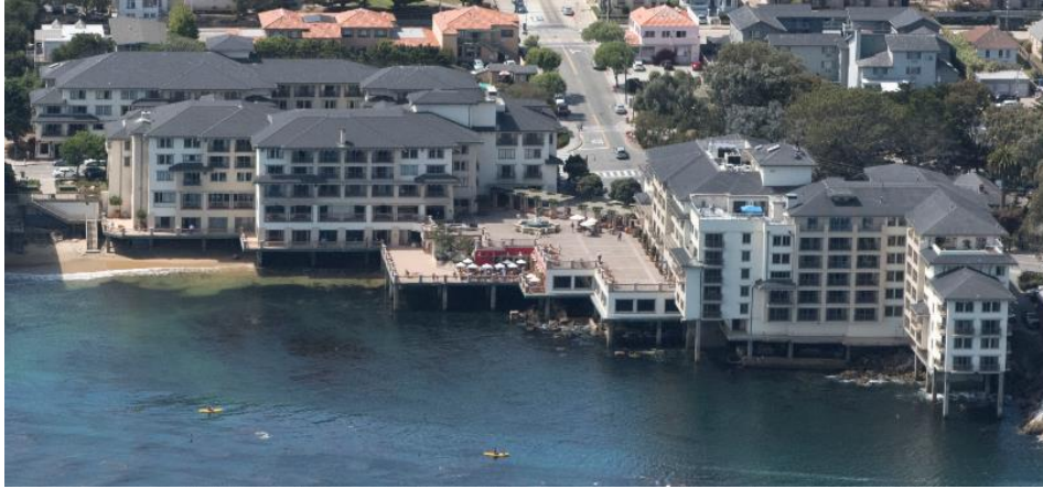
Figure 6-2: Monterey Plaza Hotel (5-7 stories) supported on Open Pile Foundation
