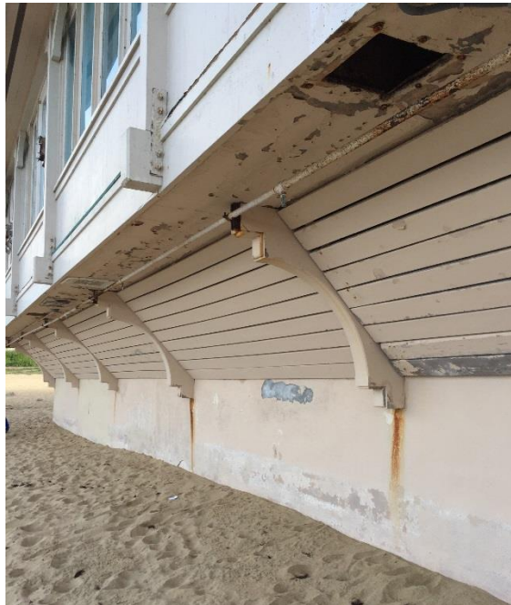
Figure 6-6: Spindrift Inn Timber Return Wall below Deck
