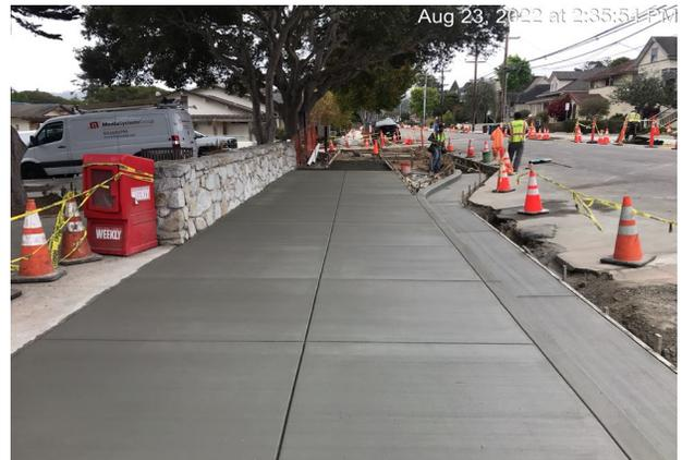
The reconstruction of Van Buren Street also included replacing the concrete curb, gutter and sidewalk along portions of Van Buren Street.
