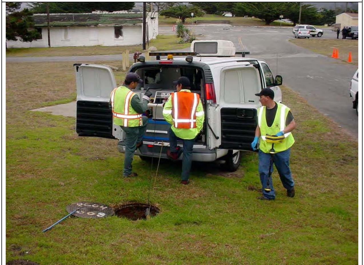
Recording Video and Physical Location of Sewer Lines in the Lower Presidio
