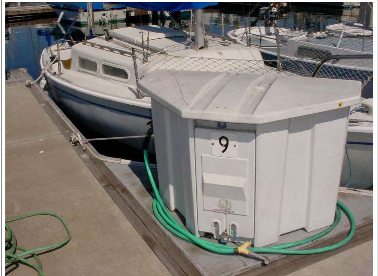
A typical dock box with electrical connections.
