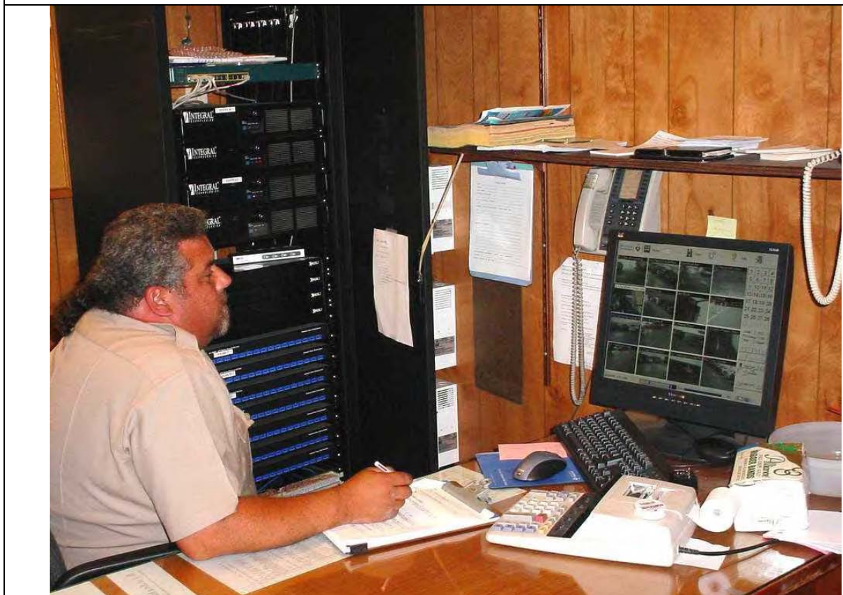
A parking technician monitors the cameras in the control room Behind him are the DVR recorders and camera hubs
