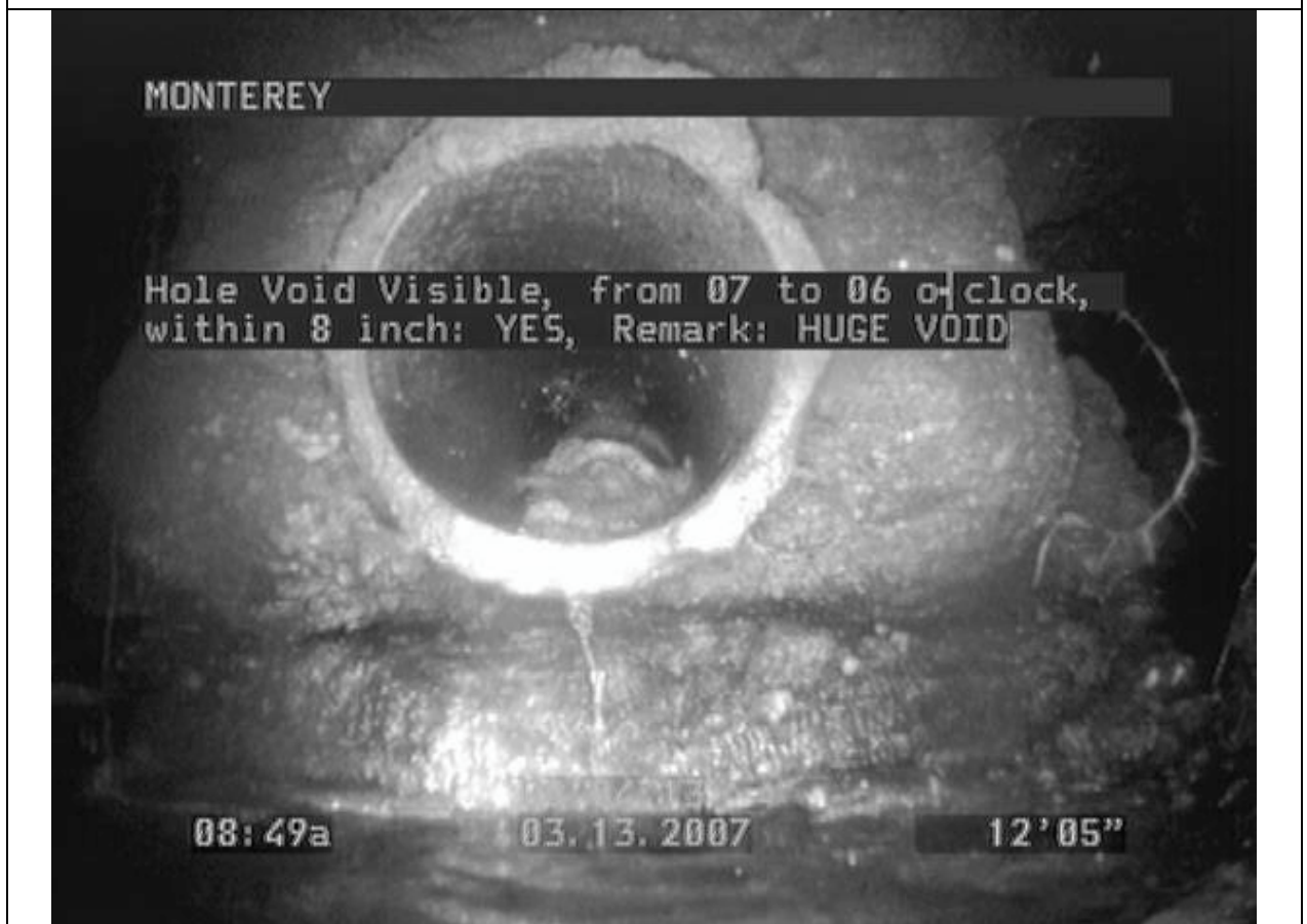
A Sewer Main Void Under Laine Street
