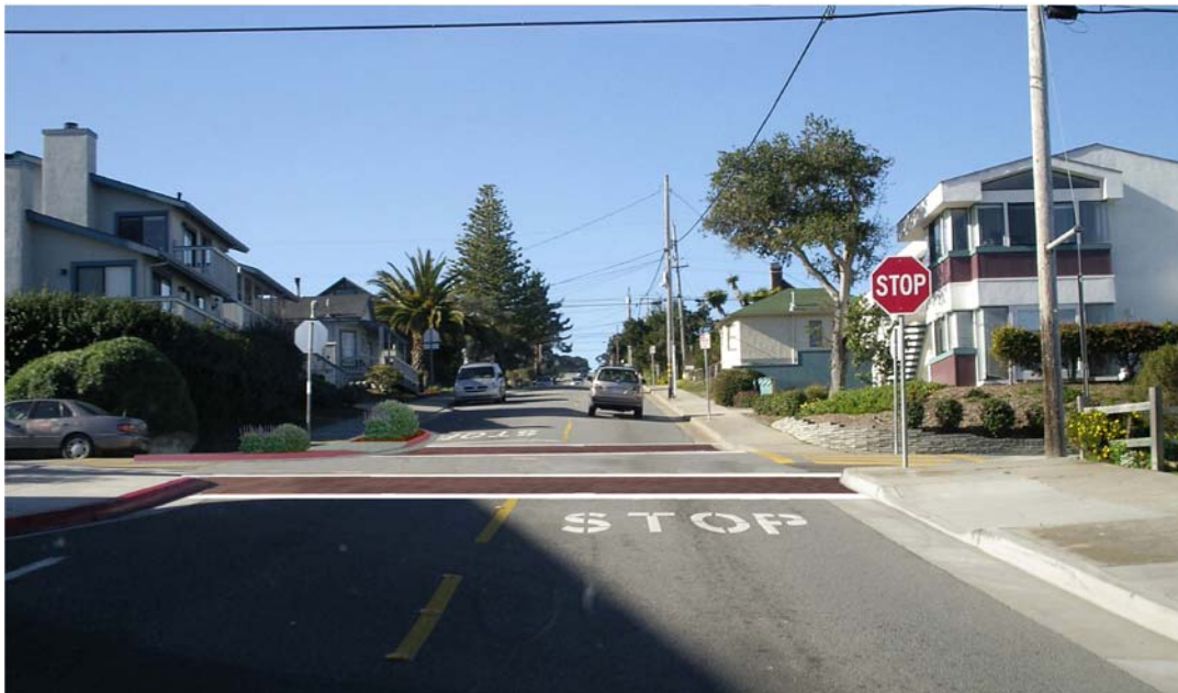
Figure 3: Rendering of Curb Extensions with Pedestrian Crossing Treatment on Prescott Avenue at Belden
