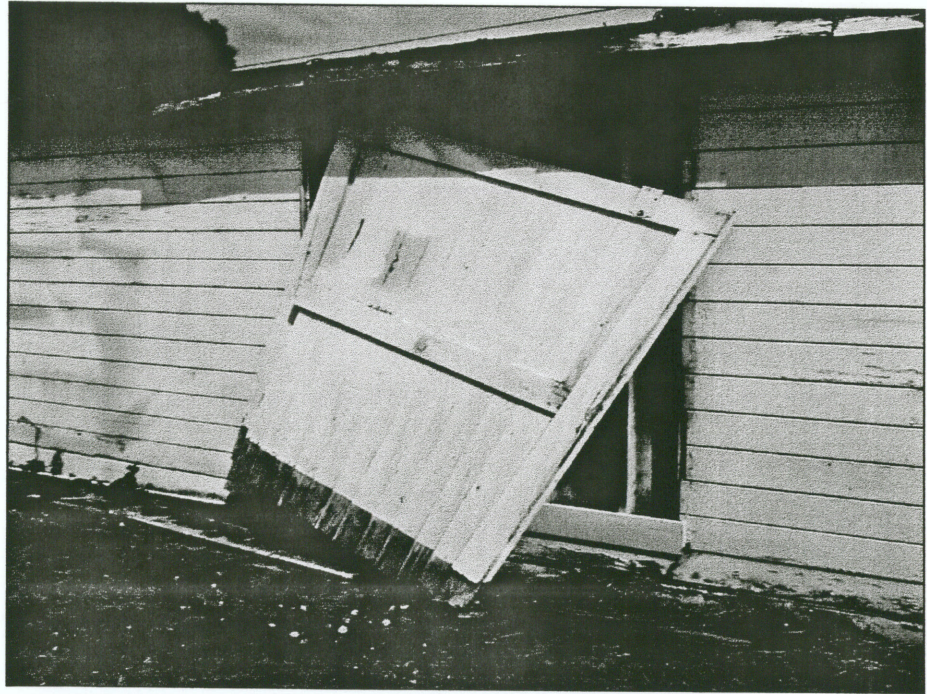
Figure 10: View of the west building from the east showing one of the sliding doors and its condition. These doors have been reused, but may have been also part of the stable period. See Figure 1 for the two sliding doors indicated on the plan. This specific door appears to be in the same location.
